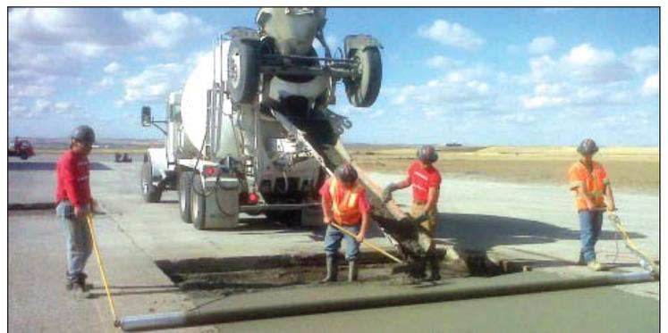
**PHOTO: Construction crew pours new North Ramp concrete.** Port file photo.
